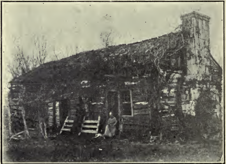
This old building, which is a double log house with two large outside chimneys, has an open fireplace in which logs of wood were burned. Was erected about 1833 when the Seneca and Cayuga Indians of New York were located here. This building was still in use as the U. S. Indian Agent's headquarters when the Modoc prisoners were brought to Quapaw Agency in 1873.
