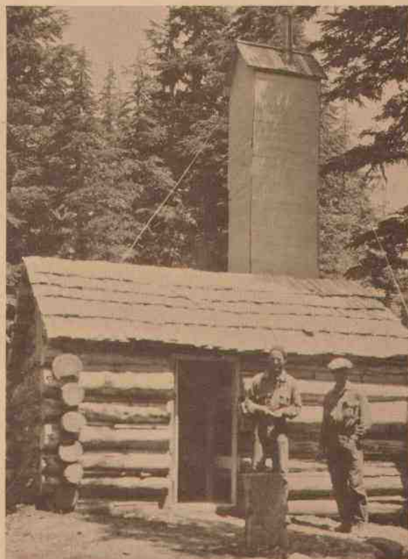
IV-14. Snow survey cabin built in about 1930 at South Lake (Seven Lakes Basin) by the Soil Conservation Service. Note the enclosed entrance tower, used when the cabin was covered by drifting snow. (RRNF Collection)
