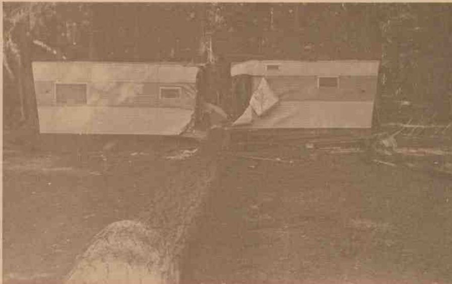
V-19. Result of "timber harvesting" by the Columbus Day windstorm, 1962. This trailer, fortunately unoccupied at the time, was located at Union Creek administrative site. (RRNF Collection)
