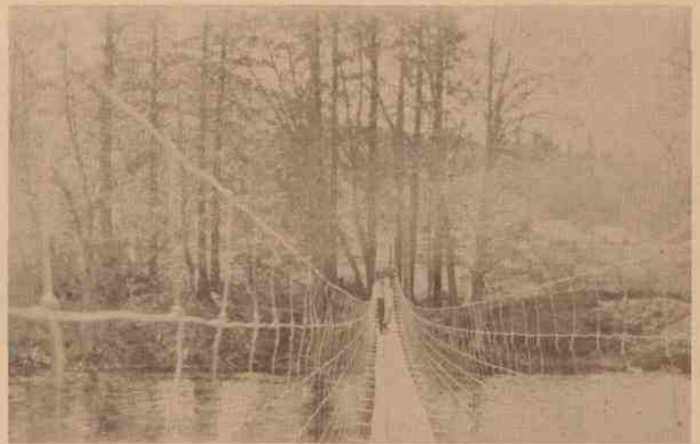
III-7. Applegate Valley settlers built suspension catwalks, or "swinging bridges" like this one, to provide access across the river, circa 1910. (Southern Oregon Historical Society)
