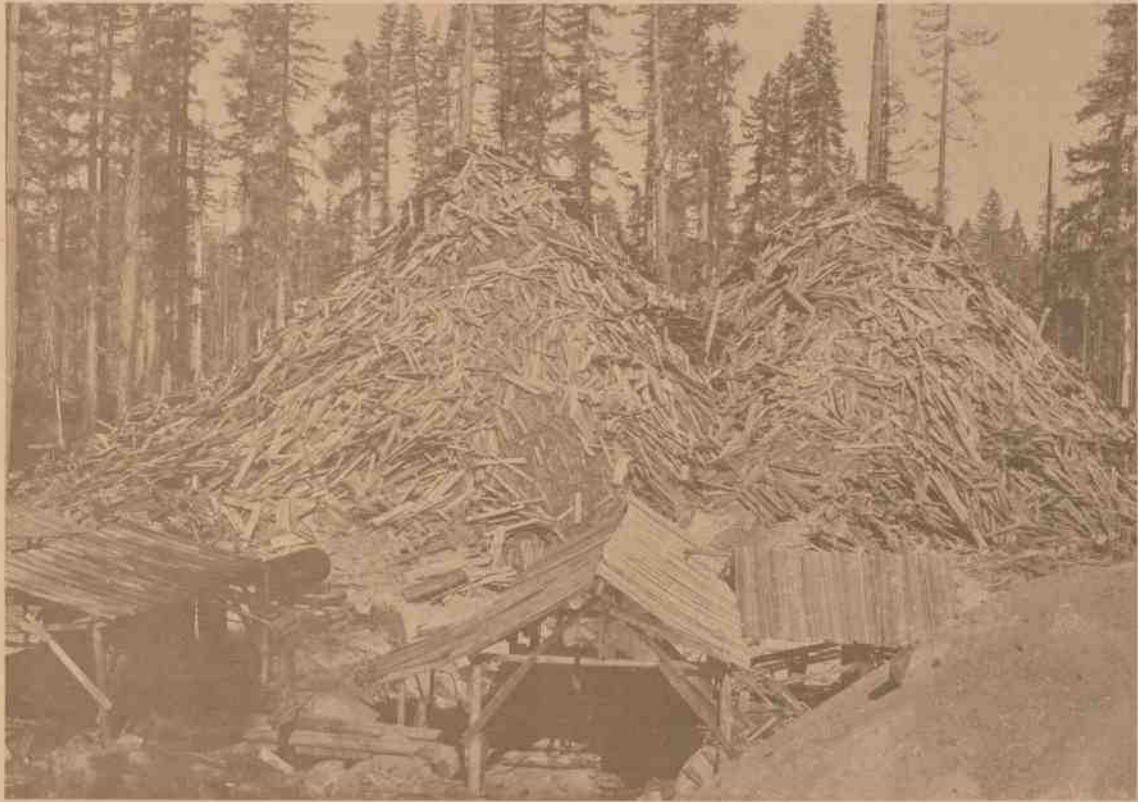
V-18. The Svindth tie mill in 1944, located near the National Forest boundary northeast of Prospect. This operation manufactured railroad ties from Douglas-fir; the two "mountains" of slab waste are about fifty feet high. (RRNF Collection)
