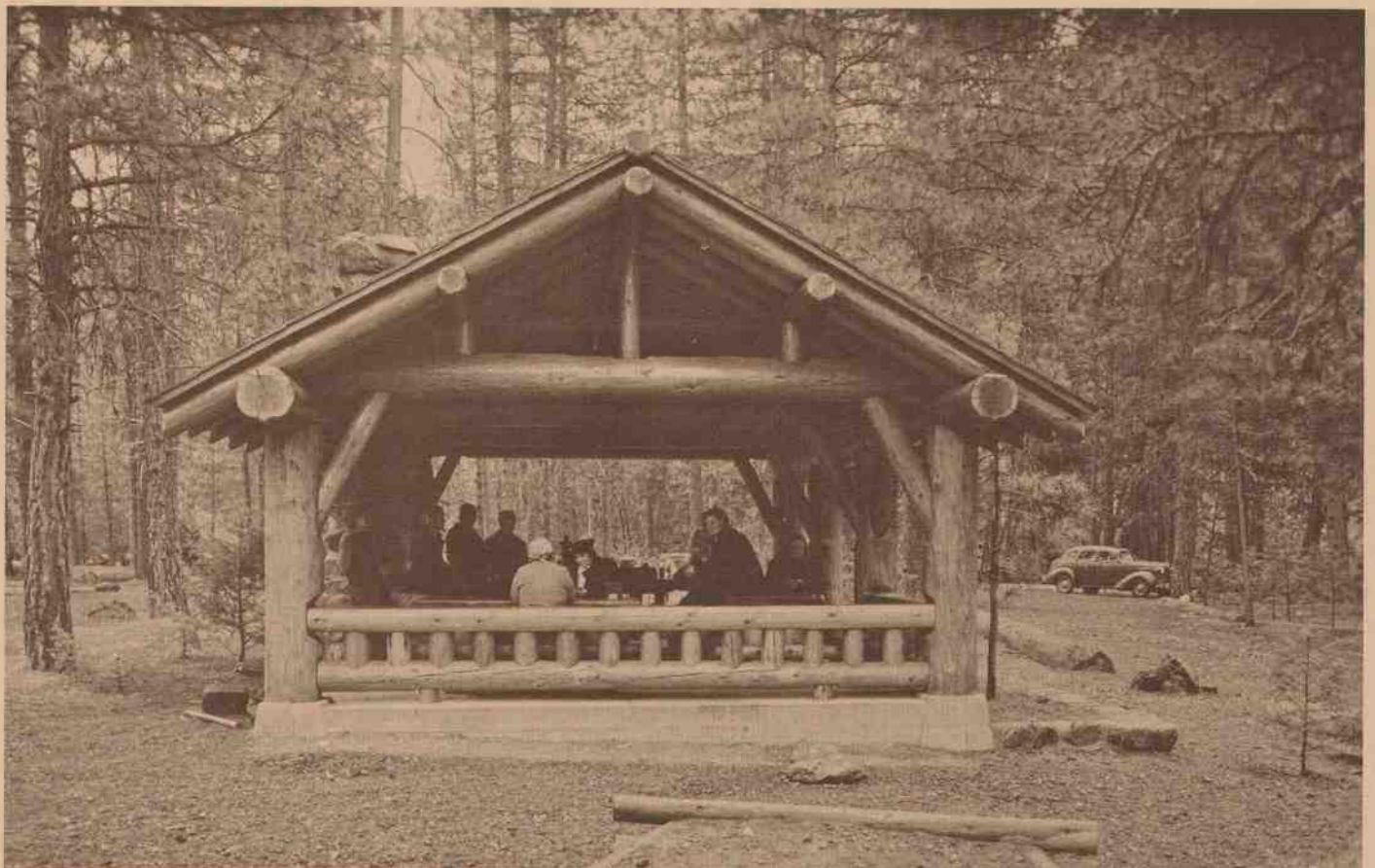
III-16. The Civilian Conservation Corps built a "community kitchen" shelter at McKee Picnic Ground, on the Applegate River. This 1936 photo shows a group of local residents preparing a picnic lunch soon after the "rustic"-style structure was completed. The only nails used in the construction held the shakes to the roof. (RRNF Collection)
