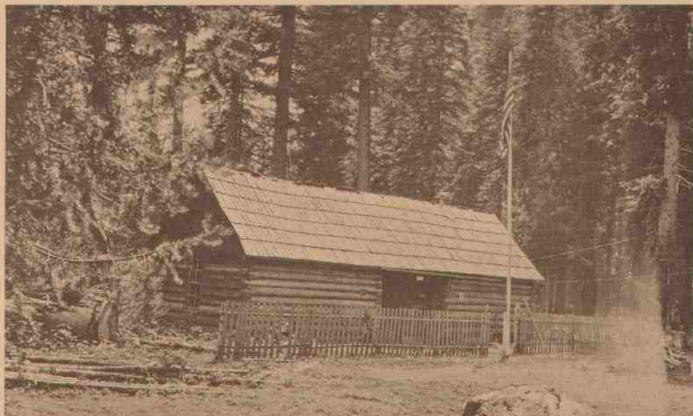
IV-12. Big Elk Guard Station, cabin constructed in 1907 — the first USFS-built structure on the National Forest. The open breeze-way ("dog-trot") between the two rooms was characteristic of cabins built in the southeastern U.S. (RRNF Collection)
