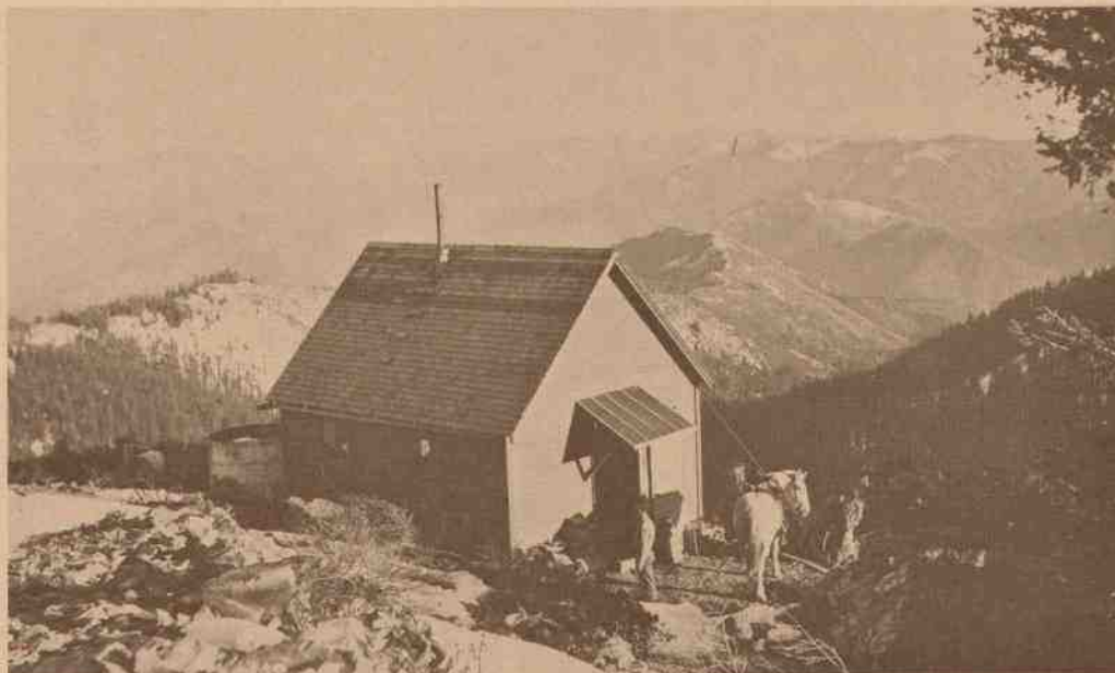
II-13. CCC-built residence at Whisky Peak Lookout, inhabited during the snowbound winters by members of the Aircraft Warning Service during World War II. (RRNF Collection)
