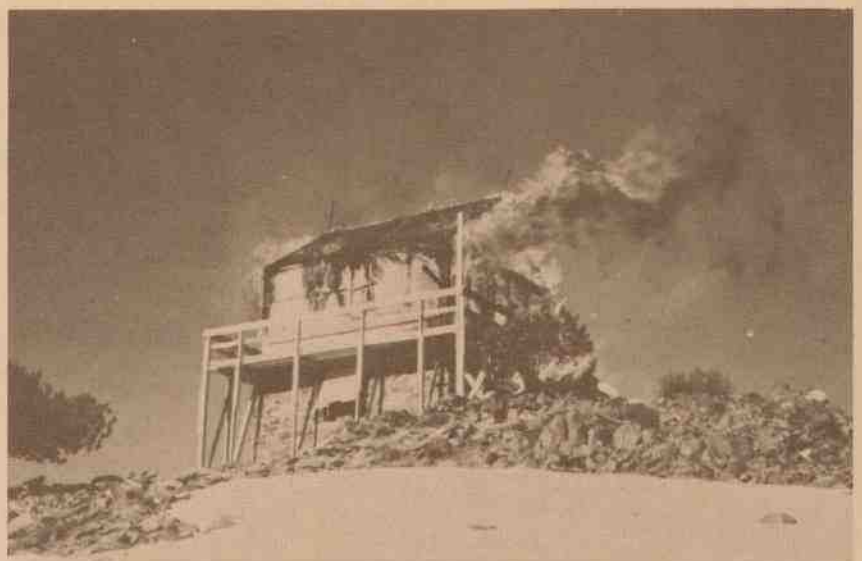
IV-19. Fire consumes Devil's Peak Lookout, circa 1968. During the 1950s and 1960s the Forest Service deactivated many of its old fire lookouts. (RRNF Collection)
