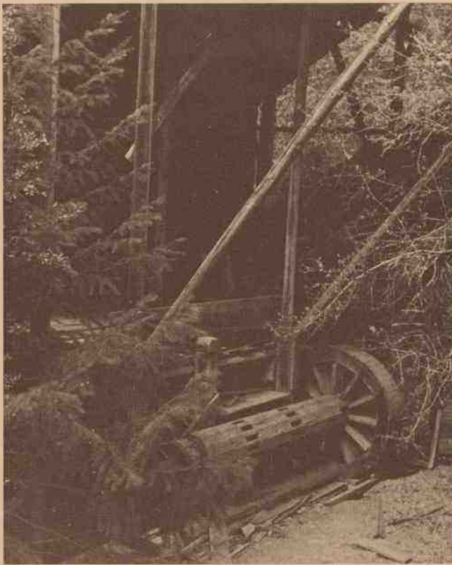
III-4. The hand-hewn wooden "bull wheel" at the now-abandoned Steamboat stamp mill, active during the early twentieth century. (RRNF Collection)
