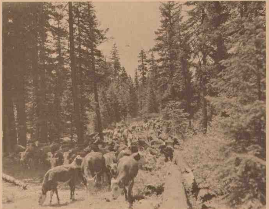
V-10. Cattle drive to the high-elevation meadows of the Upper Rogue Unit, circa 1930s. Cattle replaced sheep on the range along the Rogue-Umpqua divide during this time. Note the log drift-fence on the right, built to keep stock from straying into the nearby Union Creek recreation complex. (RRNF Collection)
