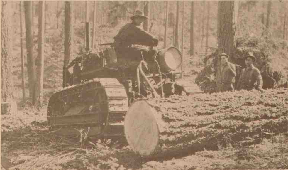
IV-10. Early-day "cat skidding" on the Fourbit Creek Timber Sale, Owen-Oregon Lumber Company, circa 1926. Hydraulic, "Robinson"-type logging arches were used with the Best and Holt tractors in order to skid the turns of pine and fir logs to the landing. (RRNF Collection)
