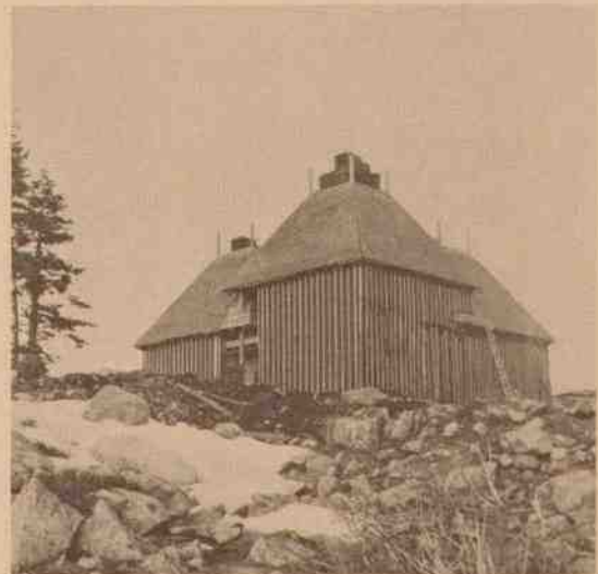
III-18. Mount Ashland Ski Lodge, under construction in 1963. (RRNF Collection)
