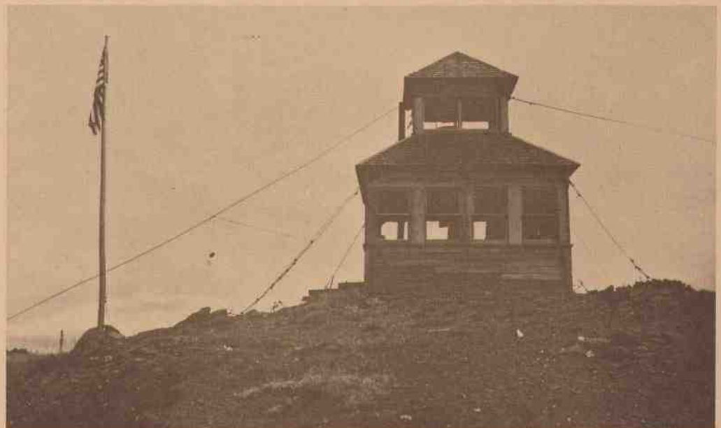
II-10. Windy Peak Lookout, a cupola-style structure built in 1914, said to be the first such building in USFS Region Six. (RRNF Collection)
