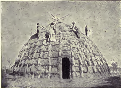
OMAHA GRASS HOUSE IN PROCESS OF CONSTRUCTION. (MOONEY)
