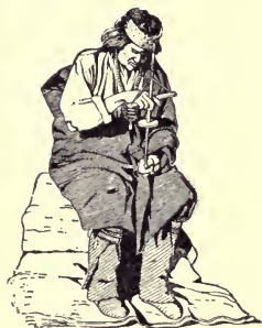
USE OF PUMP DRILL BY A ZUÑI
