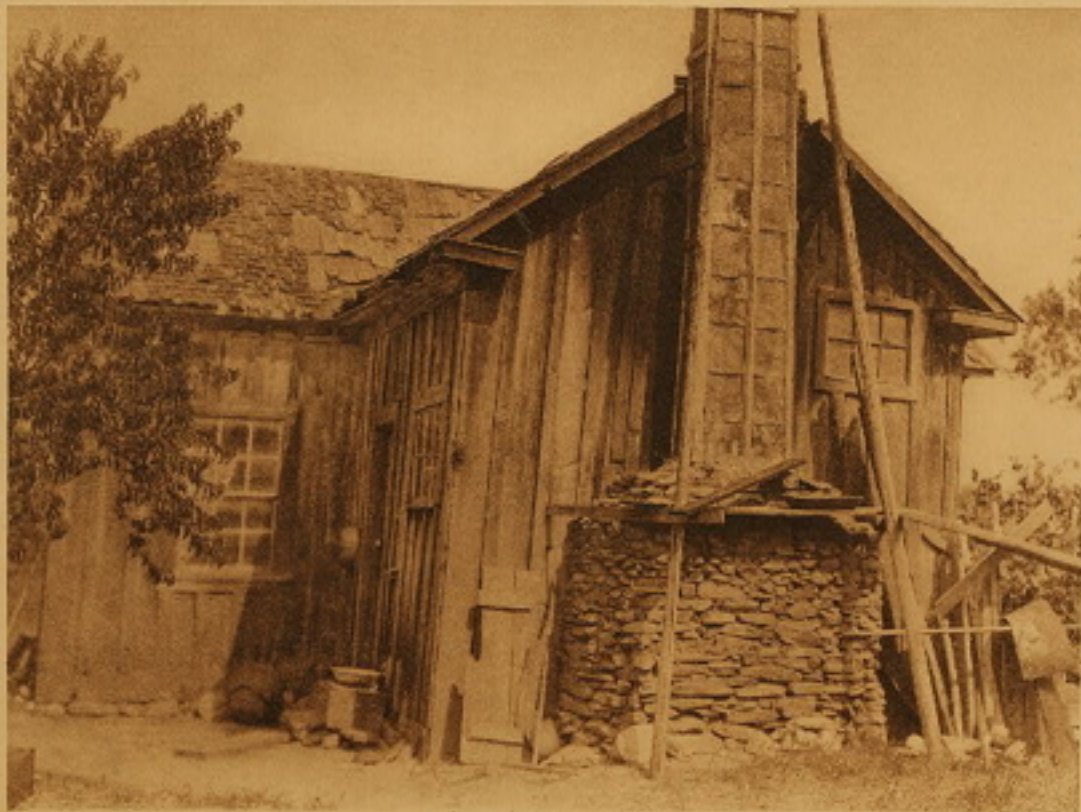
Stone Mill, near the mill, 1875, by A. P. Smith
