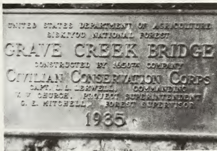
Grave Creek Bridge Plaque, 1935
